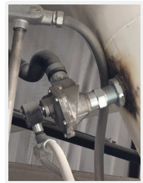
VA-12 Airsweeps® installed on the first bin for initial trial
